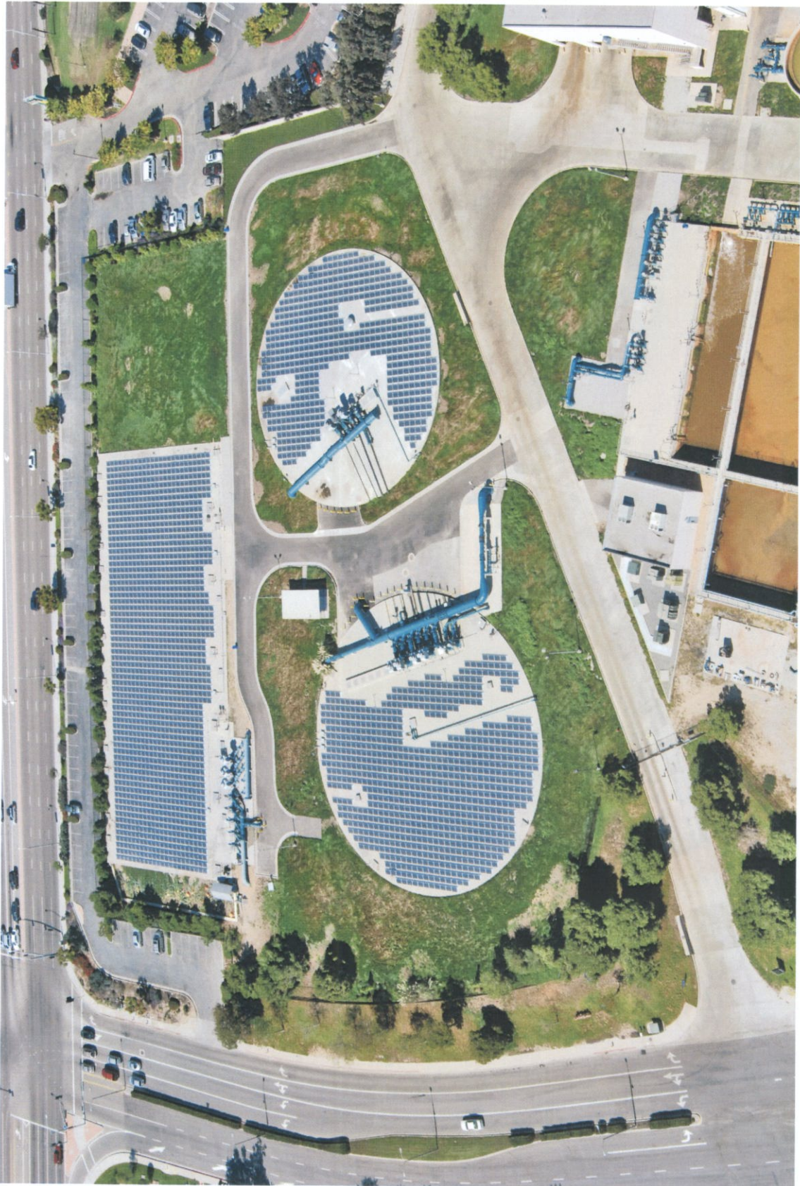
EXHIBIT "D" – AFTER INSTALLATION PHOTOS
