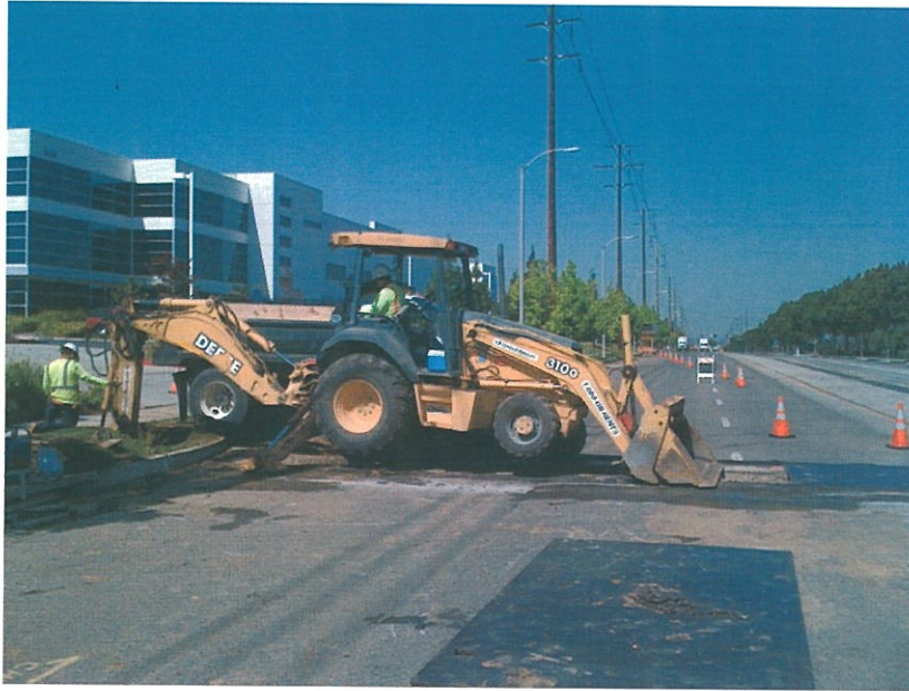
Recycled water distribution pipeline installation at Victoria and Bishop.
