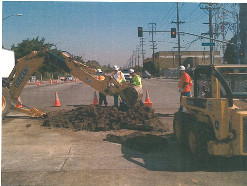
Recycled water distribution pipeline installation at Victoria and Central.
