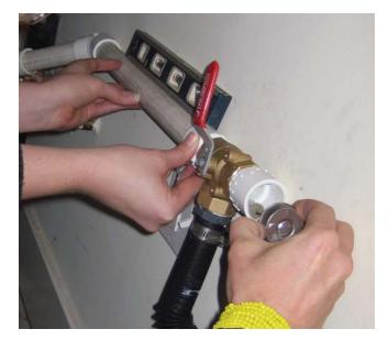
Gluing pipes on either side of a 3-way valve. Photo: Laura Allen.
