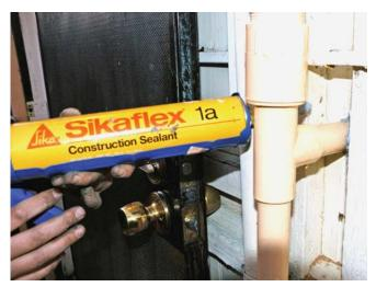
Exposed PVC pipe is painted to protect it from UV degredation. The hole is sealed with an adhesive sealant to prevent moisture from entering. Photo: David Glover.
