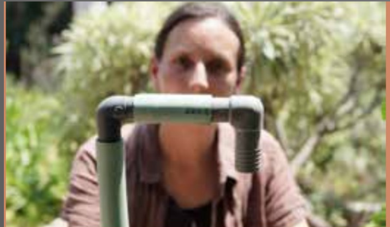
SECOND OPTION FOR OPEN END OF 1" LINE
