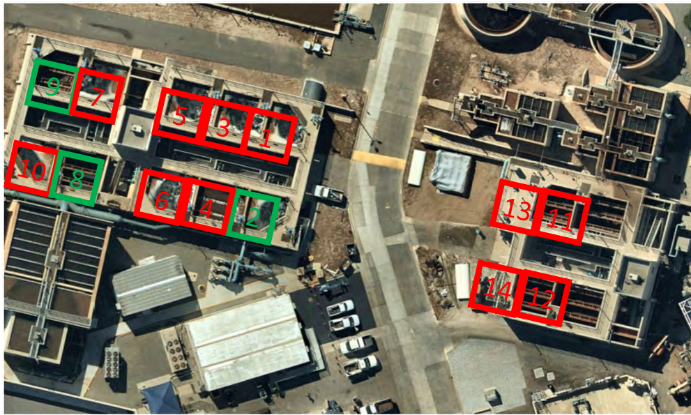
Filters 1-10 (left) and Filters 11-14 (right)
