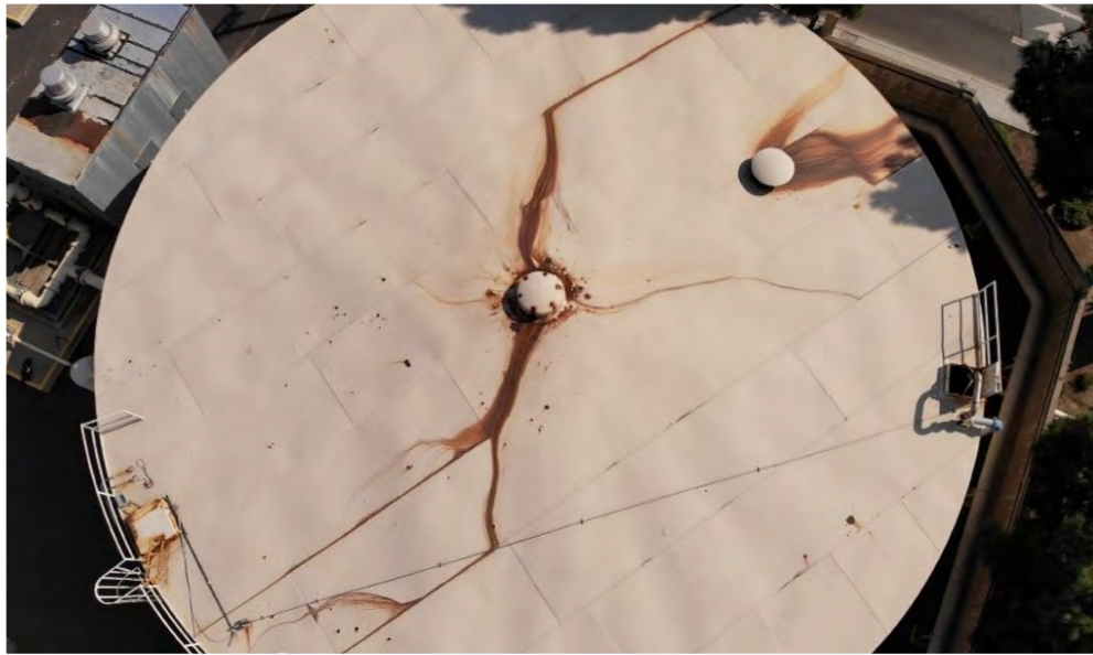
Roof of 650,000-gal steel tank
