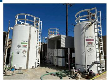
2,375-gal sodium bisulfite tanks at CNTP
